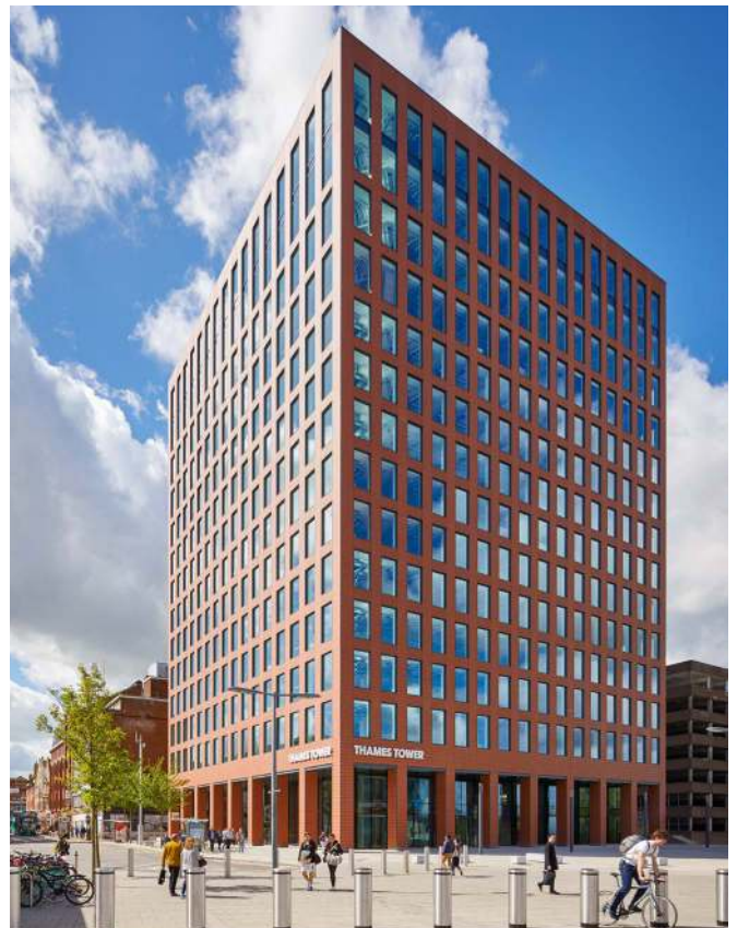
Thames Tower, Reading
