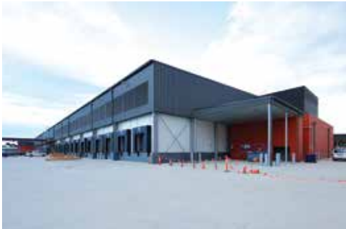
ALDI REGENCY PARK DISTRIBUTION CENTRE SA (P6)
