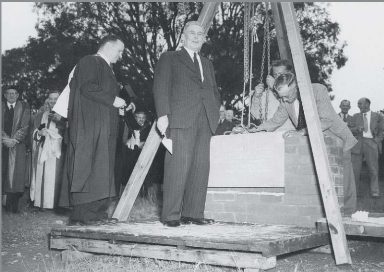
Ben Chifley, Prime Minister of Australia, accompanied by Professor Brian B Lewis, Professor of Architecture, University of Melbourne and ANU Architect, laying the foundation stone of the John Curtin School of Medical Research at the Australian National University.
