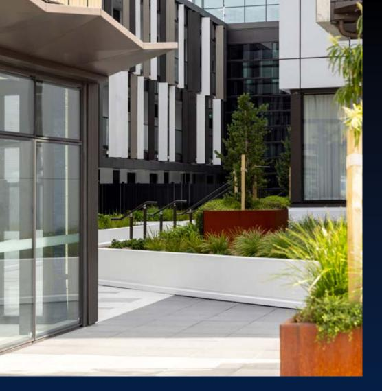
The change from rainscreen to precast façade elements, prefabricated panels and from external decks to internal Wintergardens helped drive greater cost efficiency, reduced construction time and efficiency, along with increased GFA. This improved the \$/m2 cost whilst increasing the apartment sale price potential with greater internal floor area and flexibility.
